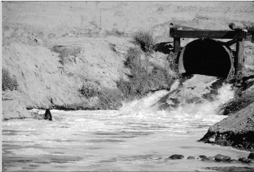
Figure 7-3 The origins of point source pollution are distinct and identifiable; hence a point source also is called an end-of-the-pipe source. Photo Barbara Tellman.
