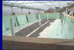
Insulation – floors and walls
