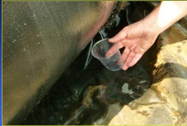
As the liquid escapes from the tube, solid particles are trapped inside.
