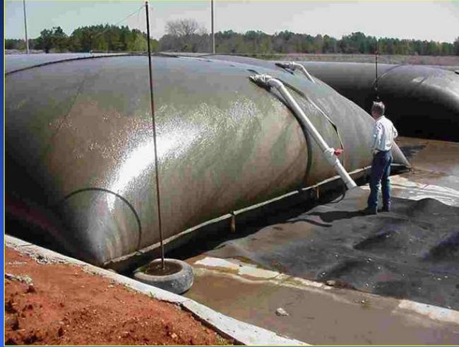
The Geotube ® is pumped with sludge material.
