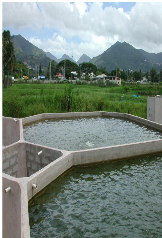
Plate 1. Octagonal concrete tanks
