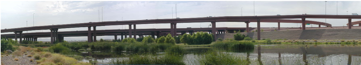
“Accidental” environmental restoration under two freeways in Maricopa County Photo courtesy of the Maricopa County Flood Control District, Arizona
