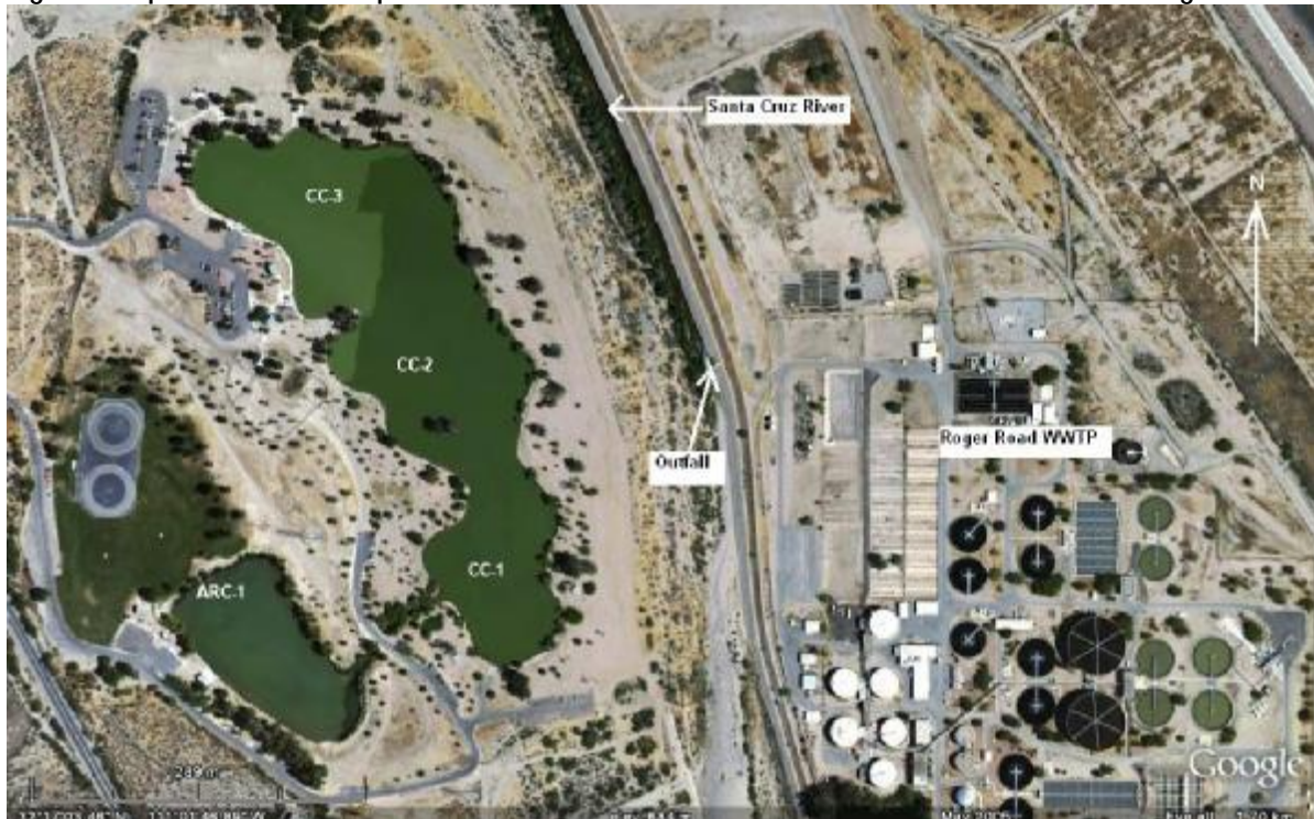
Figure 1. Spatial Relationship of CC and Archer Lakes to the Santa Cruz River and the Roger Rd. WWTP.
