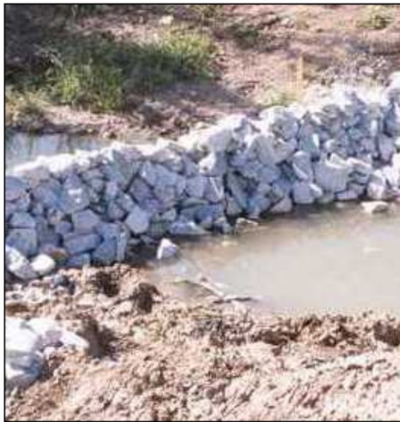
Figure 10. Check dam. Photo courtesy of ADEQ.
