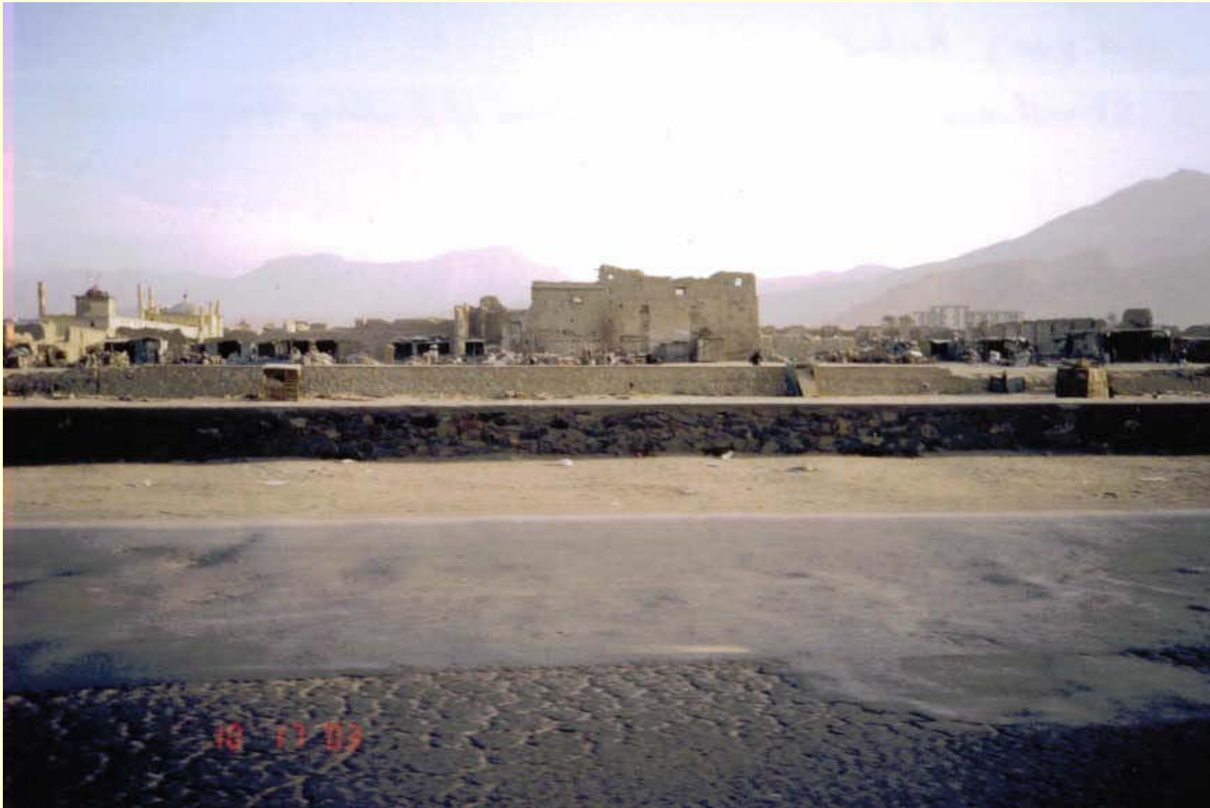
October 2003 – Kabul, Afghanistan Street scene showing evidence of building damage from war
