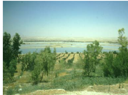
Figure 2. Khirbit As-Samra Waste Stabilization Ponds.
