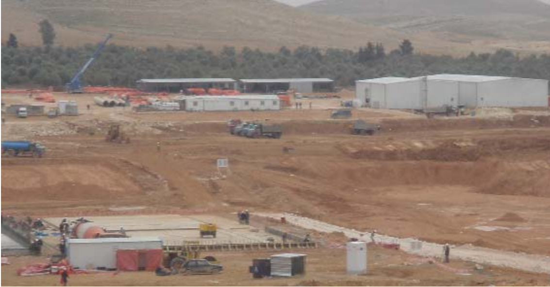
Figure 4. AsSamra WWTP Construction Site
