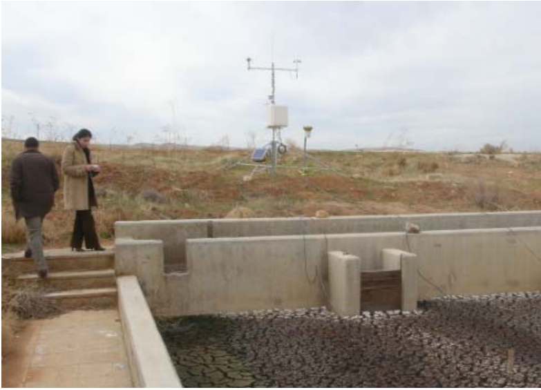
Figure 1. Experimental setup at Wadi Hassan WWTP
