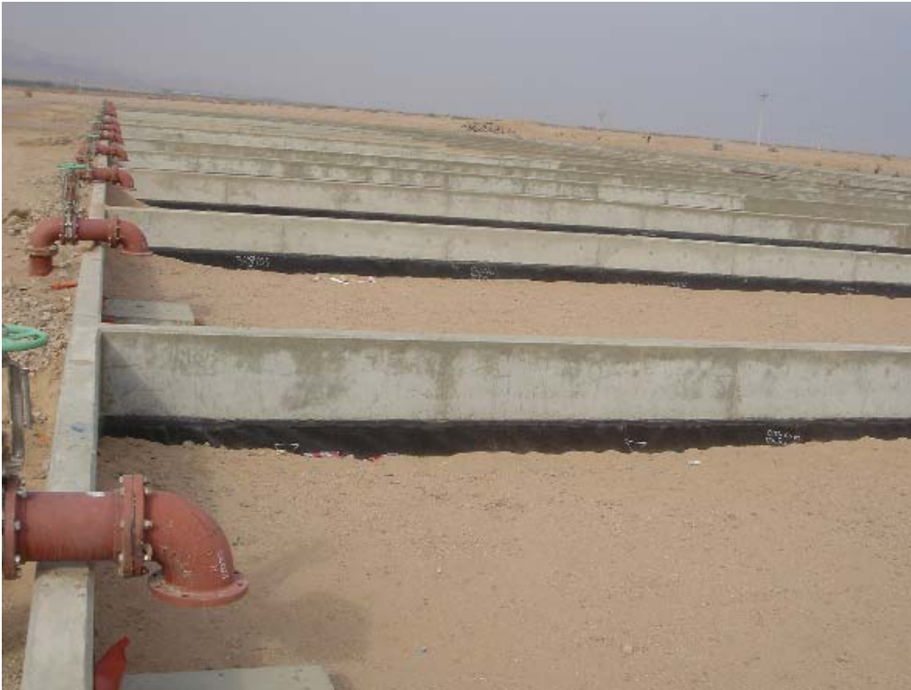
Figure 3. Biosolids Drying Beds at Aqaba WWTP
