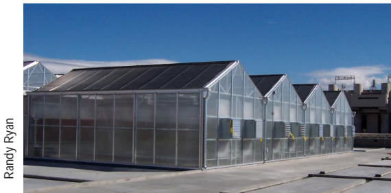
New greenhouse complex features advanced electronic controls and room to grow.
