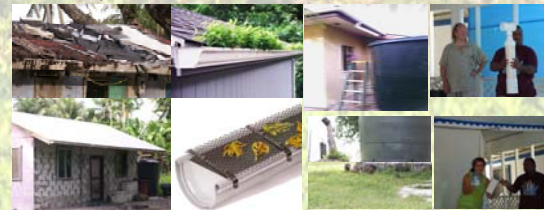
Picture 7. Views of bad and good roofs, ideal gutter, practical design for first flush diverter, and potential contaminant source for drinking water rain collection tanks and well waters (i.e. pigs).
