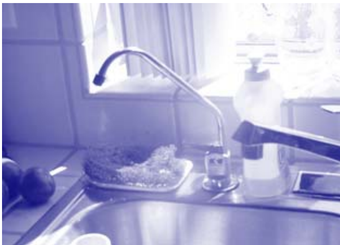
Figure 5: An example of a R/O faucet used to dispense clean water (3).
